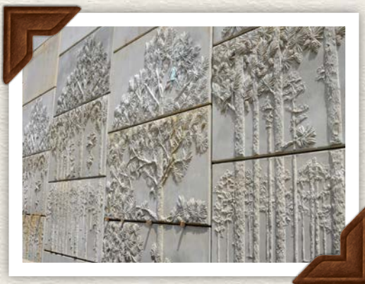
Design details of pine trees in the foundation of the Big Rock Interchange overpasses.
