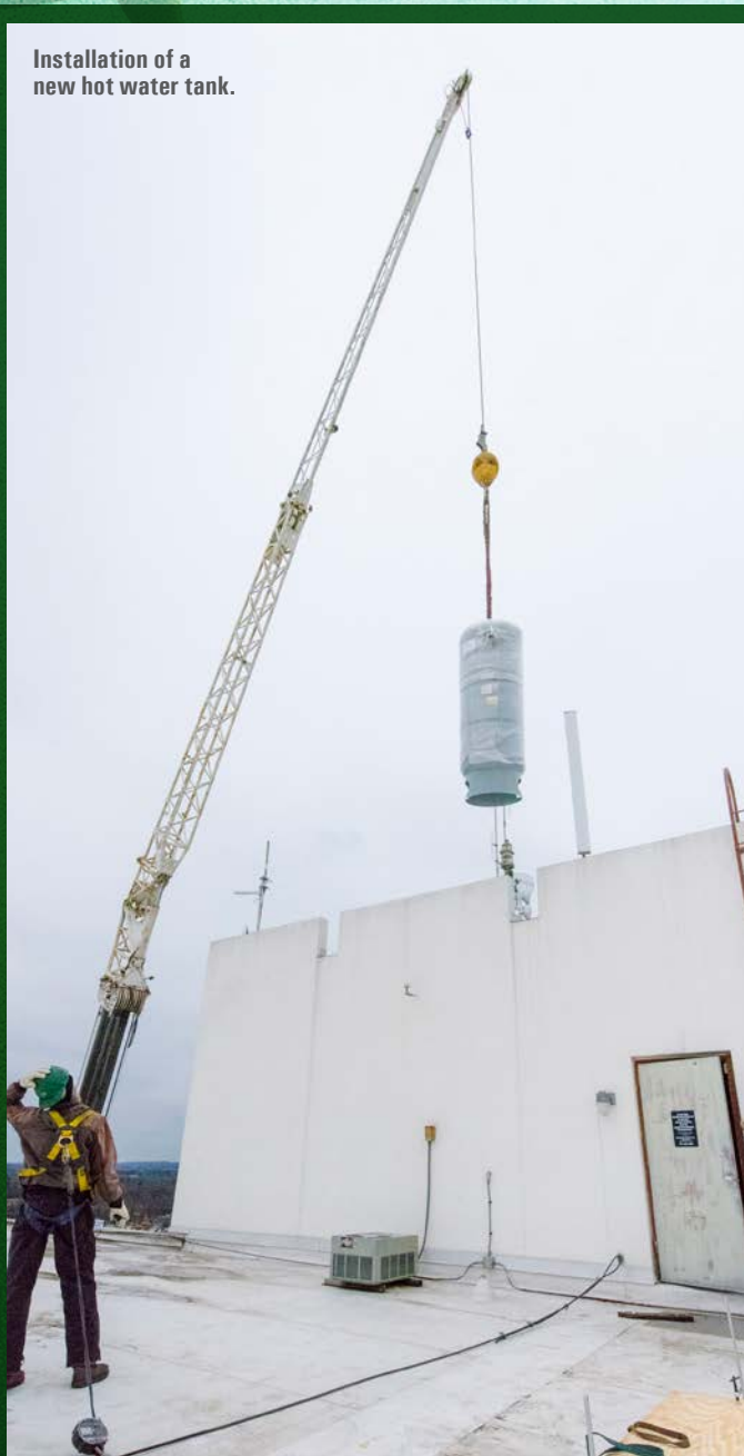
The Central Office Tower's heating system was converted from a steam boiler system to a hot water system.
