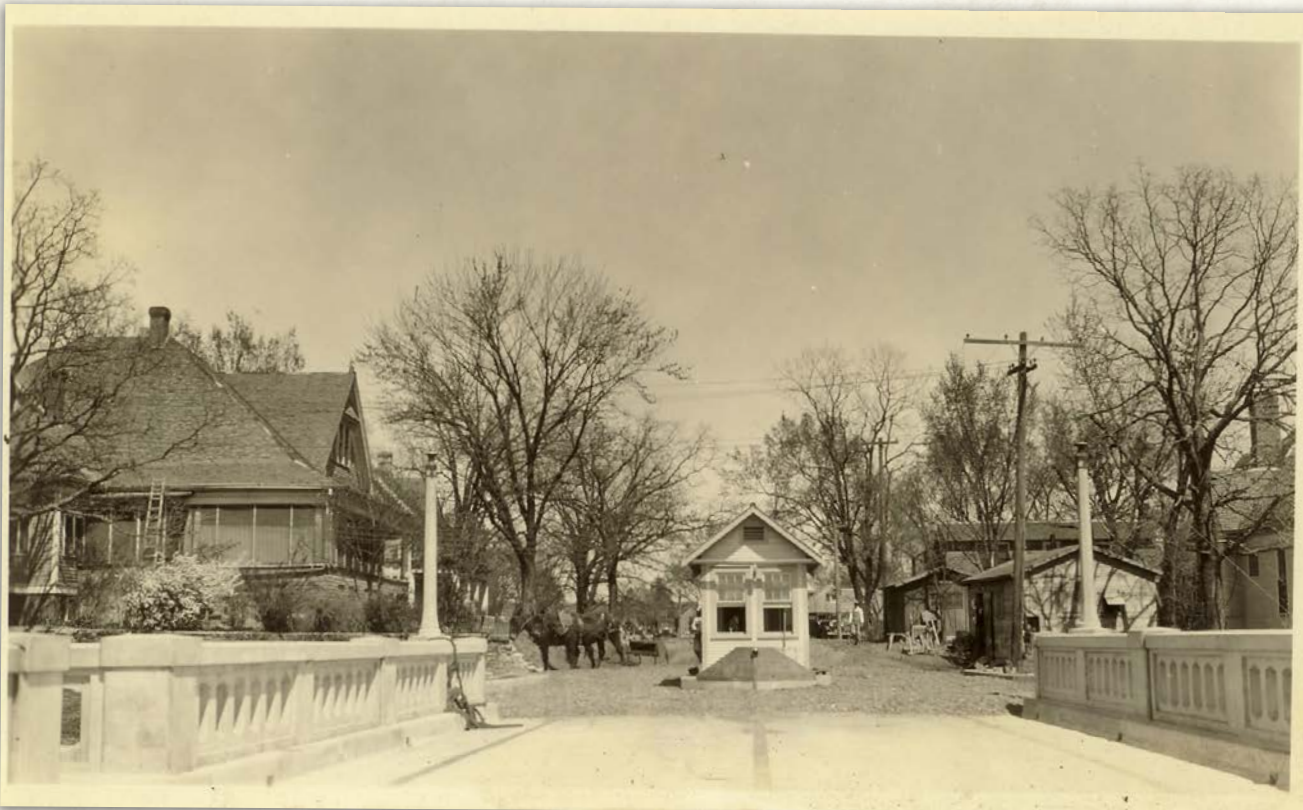
Ozark Toll Bridge Collection House, Franklin County, c. 1930
