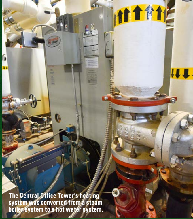
Installation of a new hot water tank.
