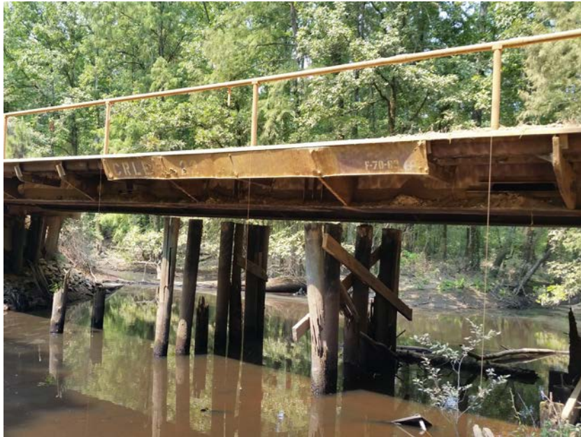
Figure 4. Little Bodcau Creek at bridge crossing (Stream 1)
