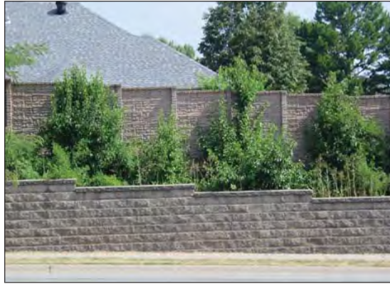
Local Example of a Noise Barrier Wall Begins at the Corner of the Intersection of Dave Ward Drive and Salem Road and Continues West along Dave Ward Drive Conway, Arkansas
