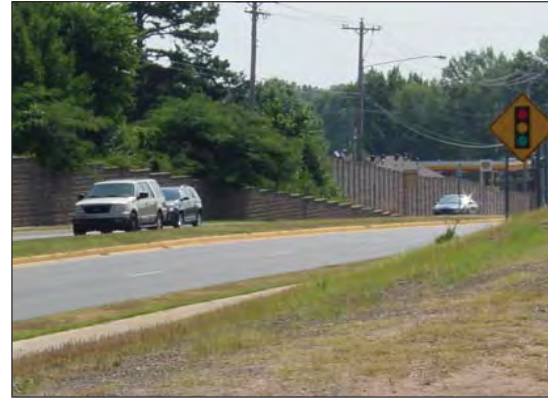
Local Example of a Noise Barrier Wall Begins at the Corner of the Intersection of Dave Ward Drive and Salem Road and Continues West along Dave Ward Drive Conway, Arkansas
