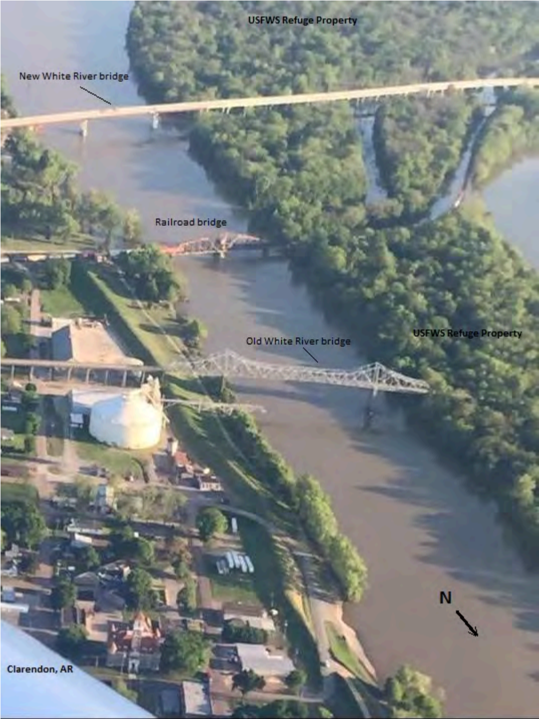
Figure 1. Project area showing newly opened Hwy 79 Bridge to the south of the old Hwy 79 White River Bridge, the Town of Clarendon to the east, and USFWS refuge property to the west.
