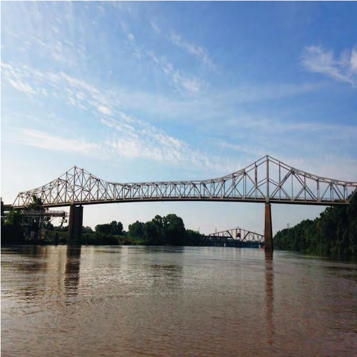
Figure 2. Main span of Old Hwy 79 White River Bridge at Clarendon, AR
