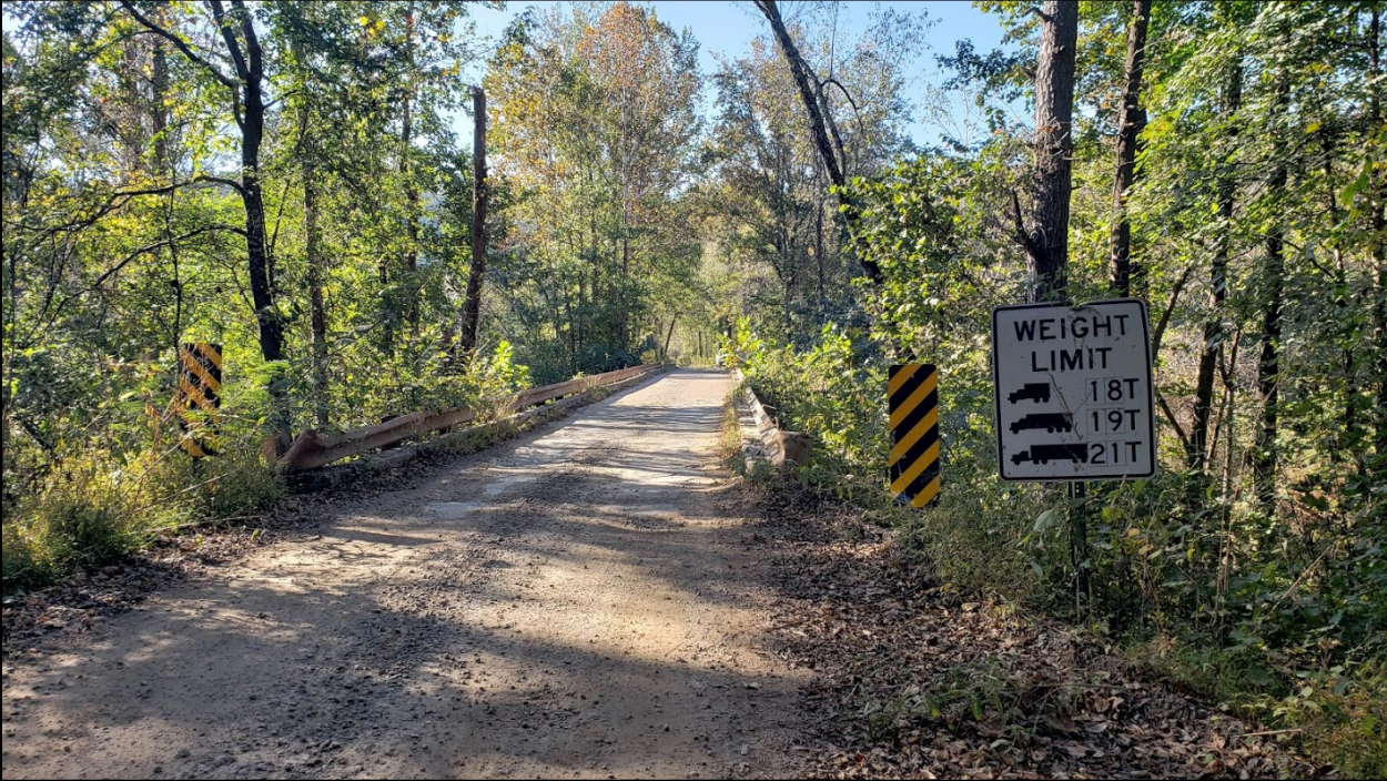
Upper View of Johnson County Road 36/5440 Bridge over Panther Creek
