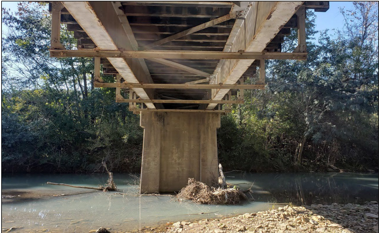
View Below of Johnson County Road 36/5440 Bridge over Panther Creek
