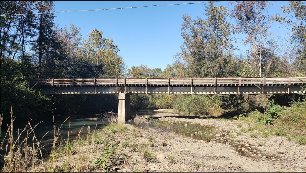
Side View of Johnson County Road 36/5440 Bridge over Panther Creek
