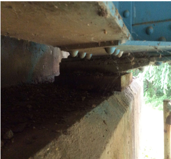
PHOTO 1 Description Bearing 1 is sitting at the edge of Cap at Abutment 1.
