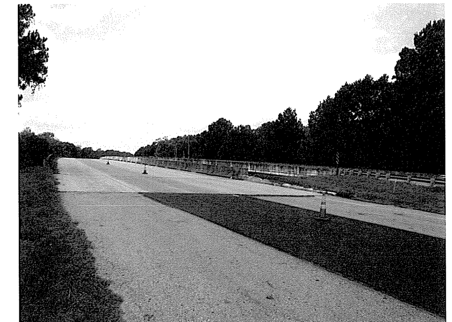
Br. A&B5791 - TOP SIDE OF BRIDGES
