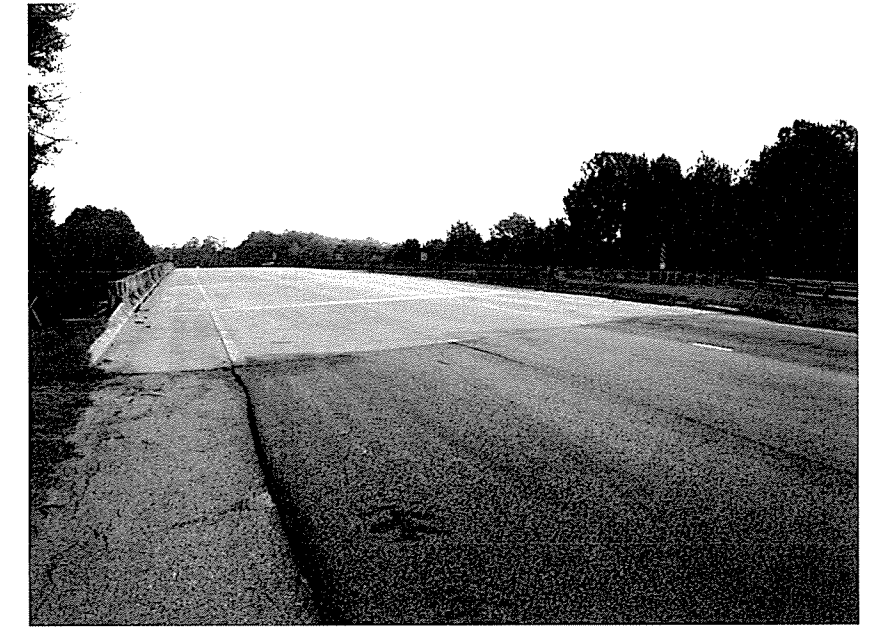
Br. A&B5789 - TOP SIDE OF BRIDGES
