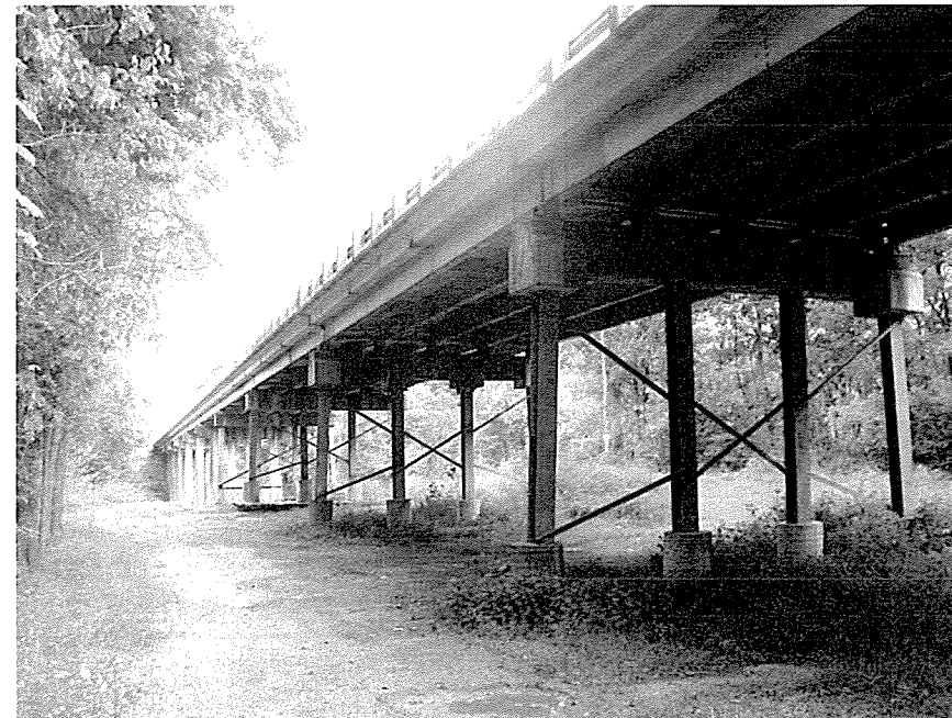
Br. 03854 - South side of bridge
