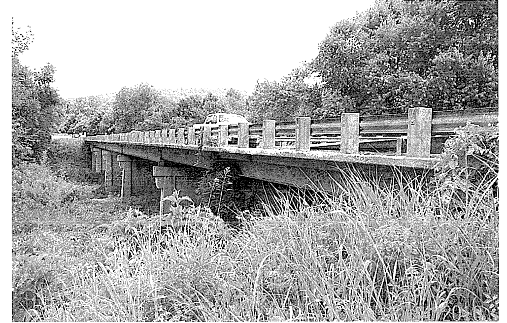
Site 3 - Bridge No. 03345
