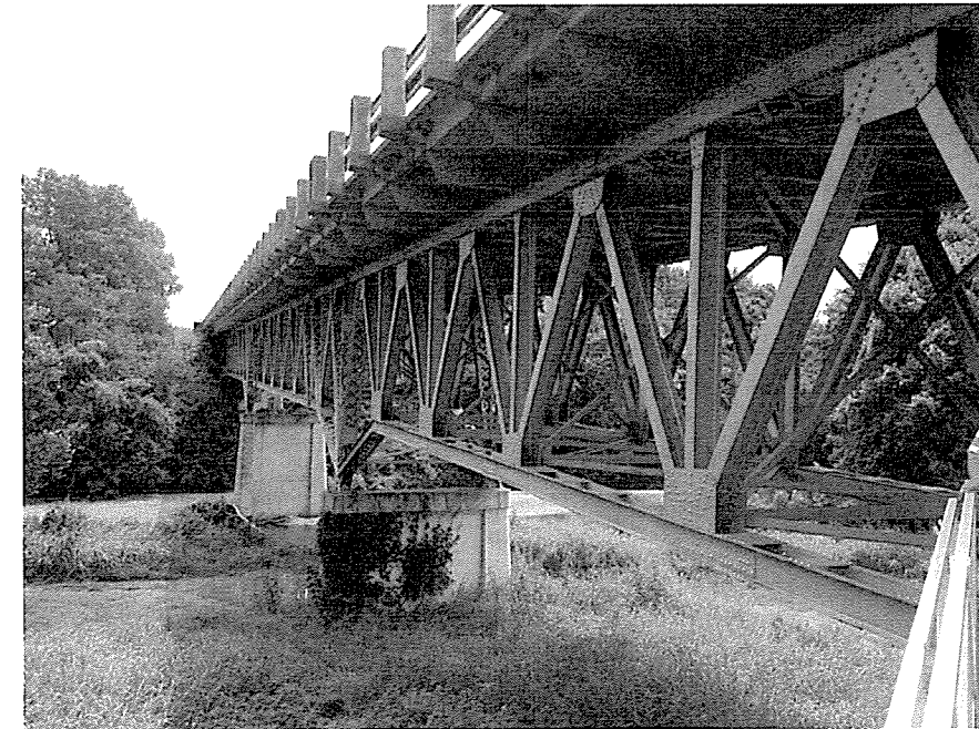
Site 10 - Bridge No. 02469
