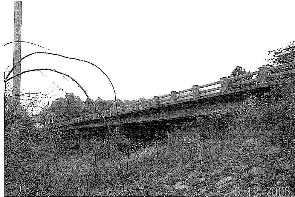
Site 5 - Bridge No. 05082
