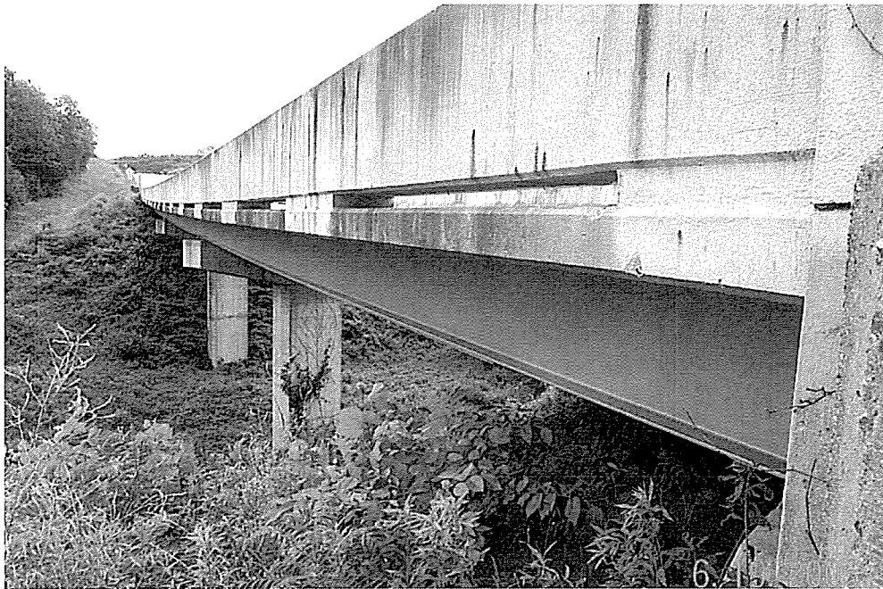
Site 4 - Bridge No. 05883
