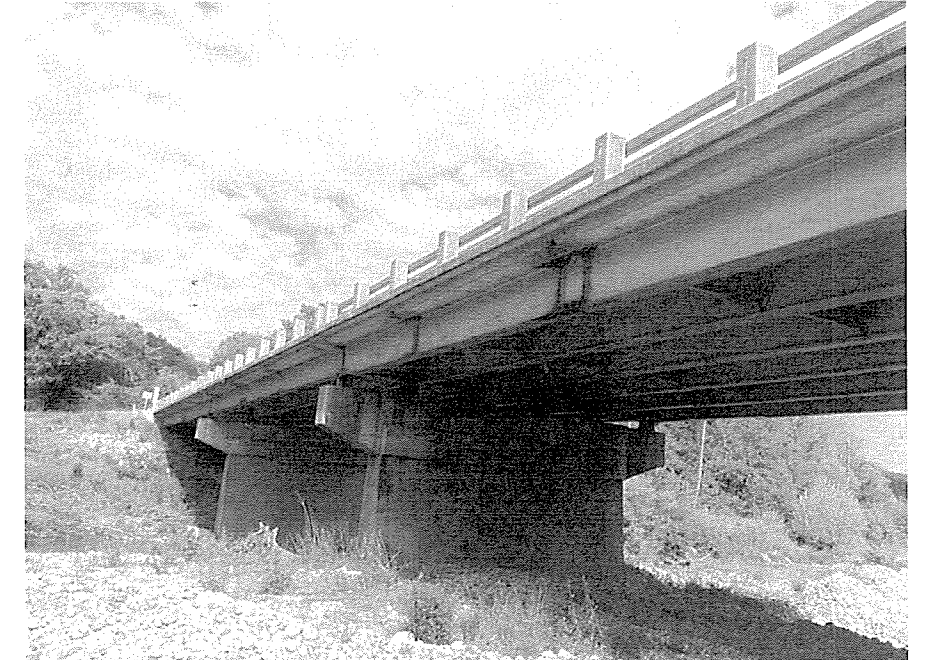
Site 6 - Bridge No. A2771
