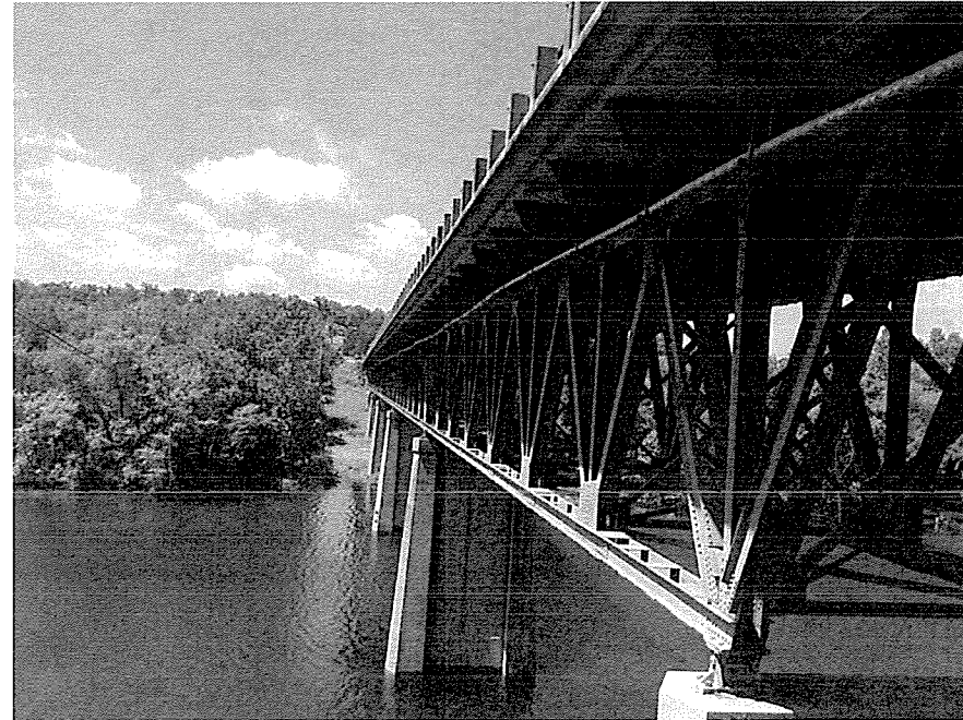
Site 2 - Bridge No. 02597
