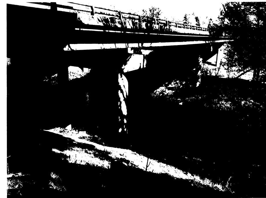
SITE NO. 6 - BRIDGE NO. A5311
