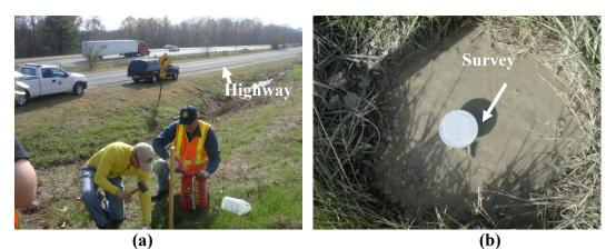
Figure 3.3. a) Installation of survey monument in the ground by UofA and AHTD personnel, and b) survey monument installed in the ground using Quickcrete®.
