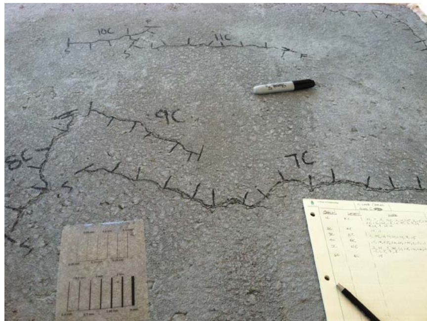
Figure 3.13 Test Slab During Crack Measurements
