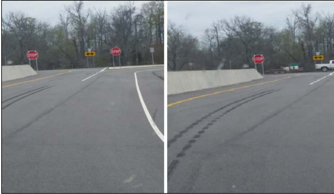
Figure A.8 STA 475 + 00
