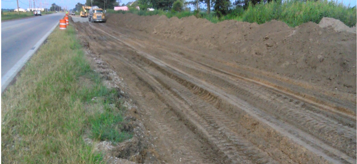
Figure 8.2 Cement Stabilization – Project 100653
