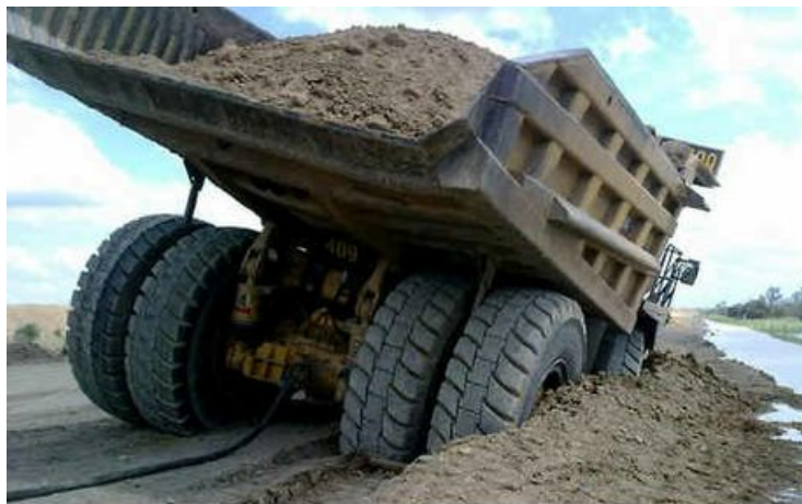
Figure 1.1 Example of Construction Operation Problem due to Soft Soil
