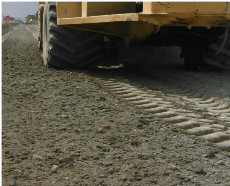
Figure 8.4 Fly Ash - Project 100653
