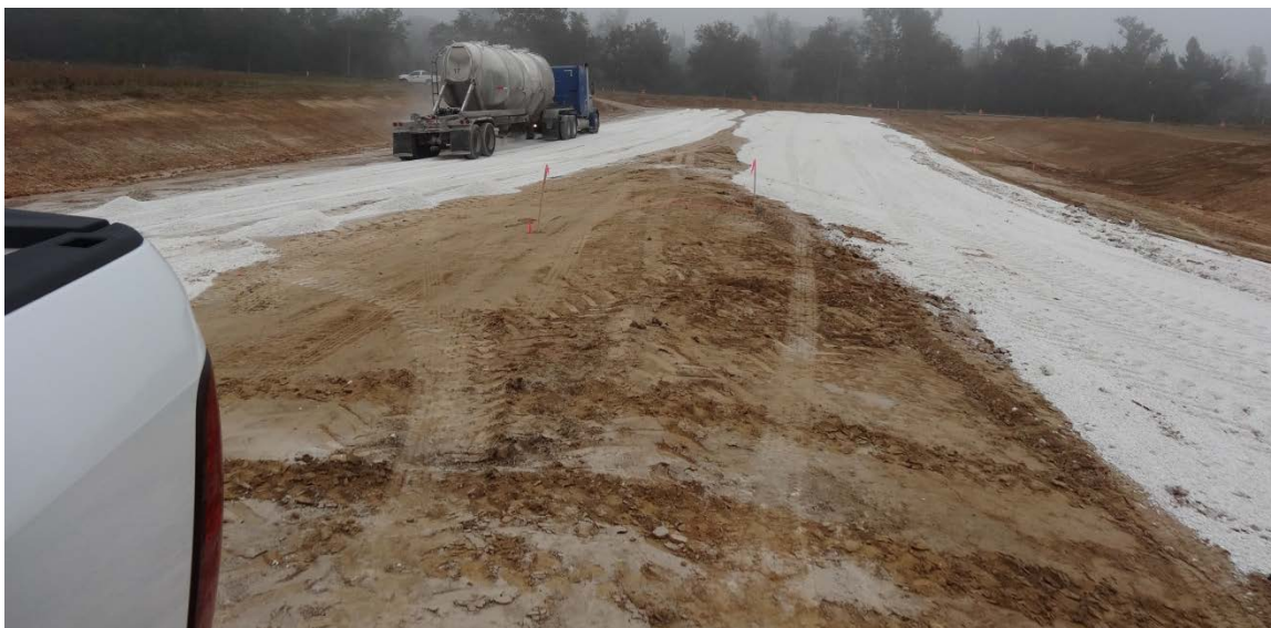
Figure 8.2 Application of Lime Stabilization – Project 060897
