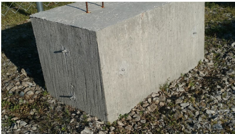
Figure 3.3.3-3: Outdoor Exposure Block (Fayetteville, Arkansas)
