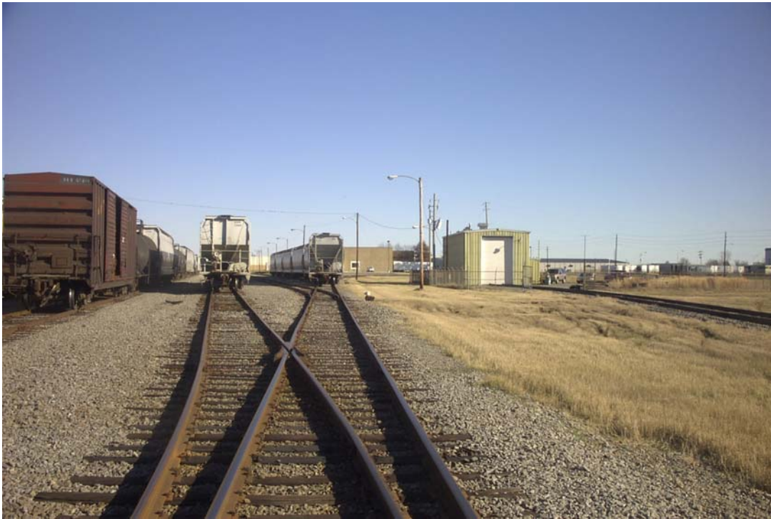
Rail Marshalling Yard
