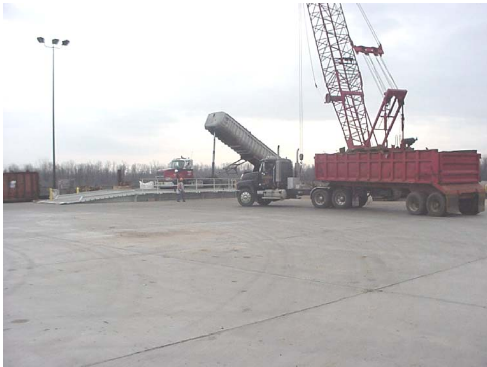
Unloading Scrap Steel at New Harbor
