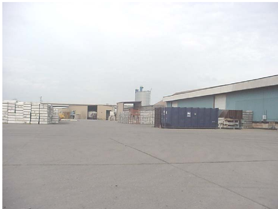
Outside Storage and Bagging Warehouse at Riverport
