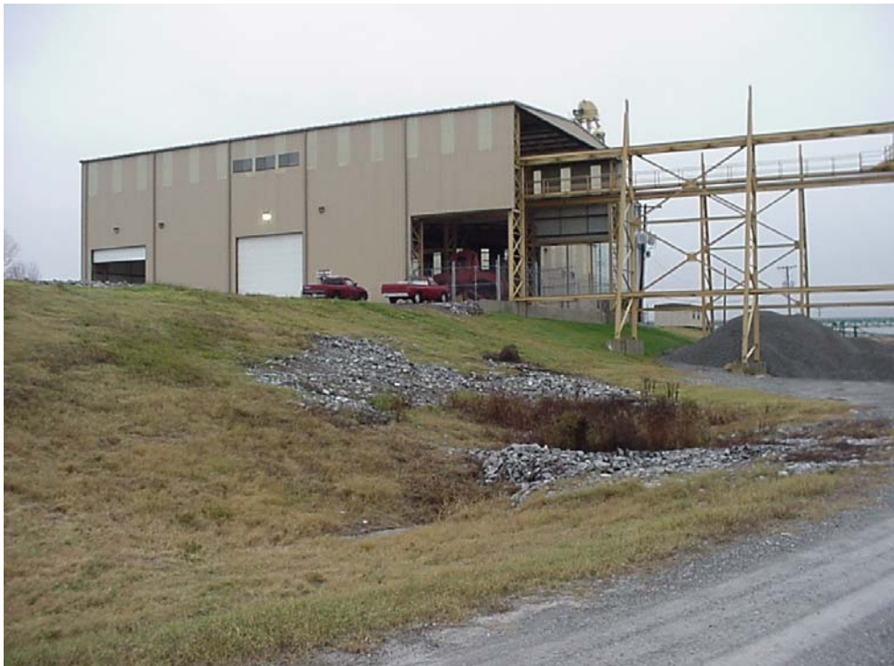
Warehouse with overhead crane
