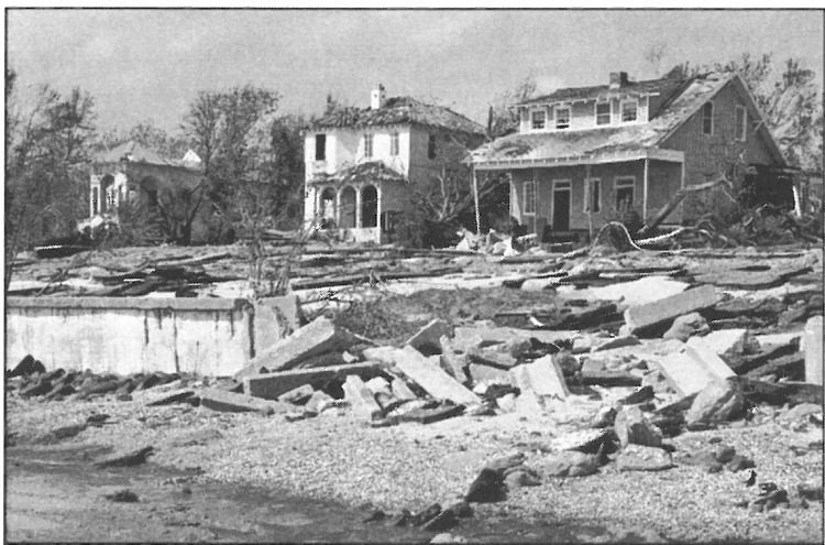
Damage to the sea wall in the Old Town area of Bay St. Louis.
