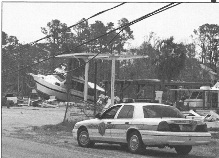
Damage in the Gulf Coast area was extensive.
