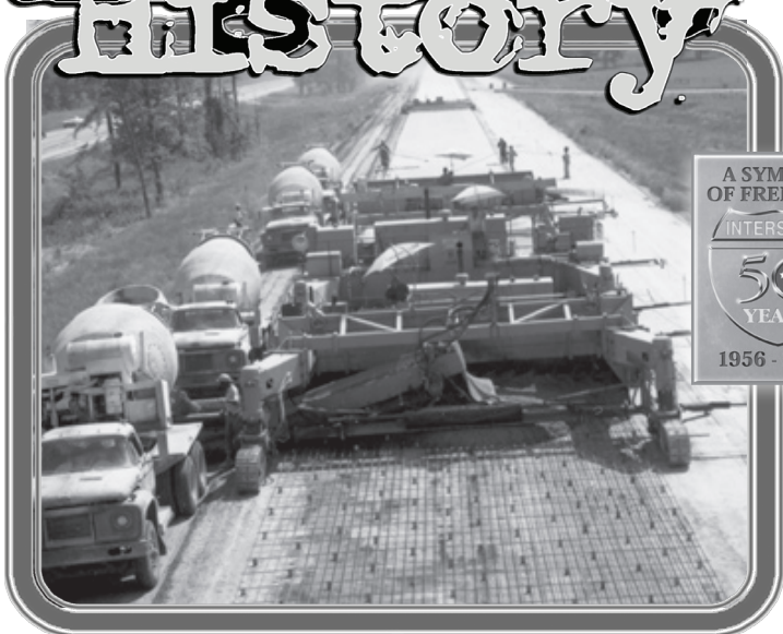
Slip form paving on Interstate 30 near Hope as seen from the Highway 4 overpass in 1970.
