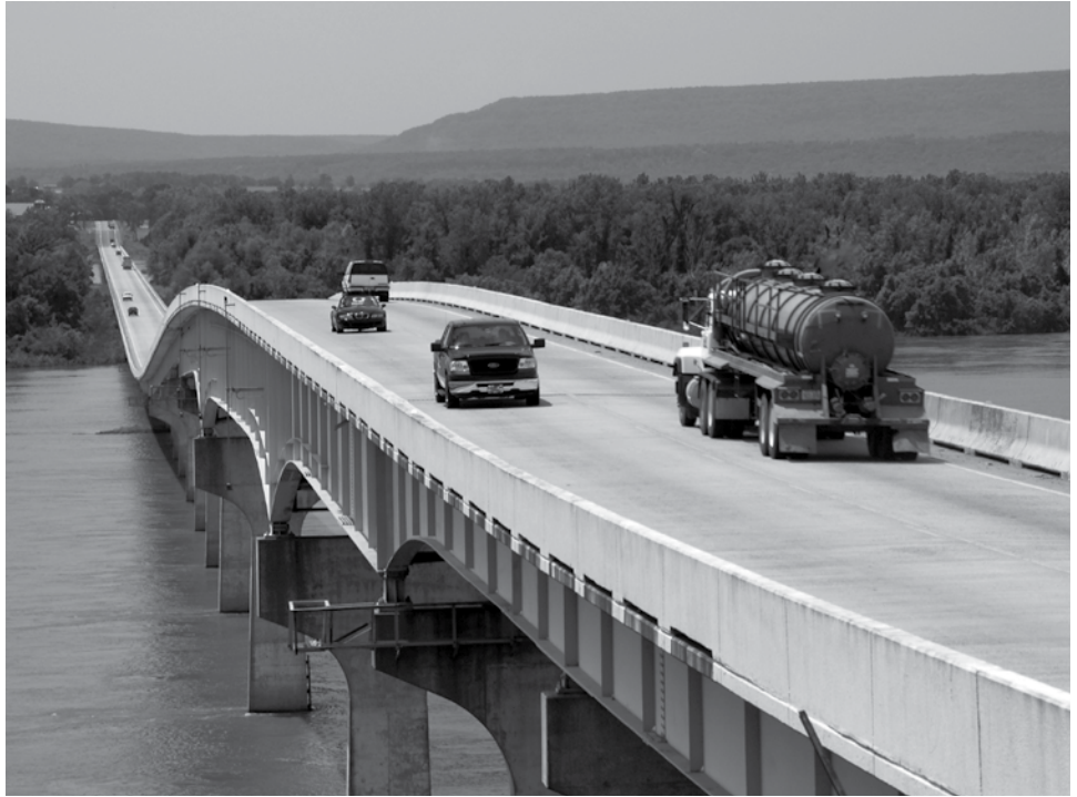
Highway 109 Bridge over the Arkansas River at Clarksville.
