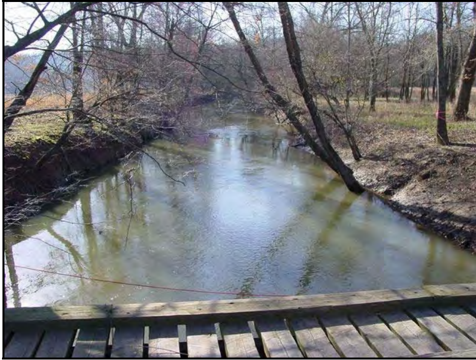
Figure 11. Bayou Des Arc at McEuen Road
