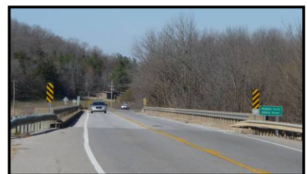
Figure 2. Existing Hwy. 16 Bridge Over the Middle Fork
