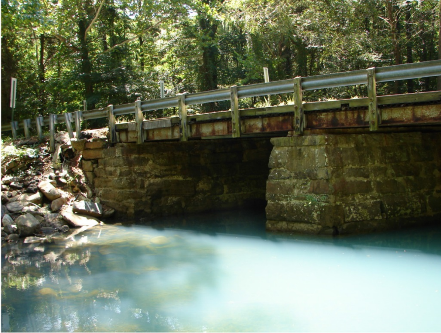
Existing Bridge with Stone Masonry Piers
