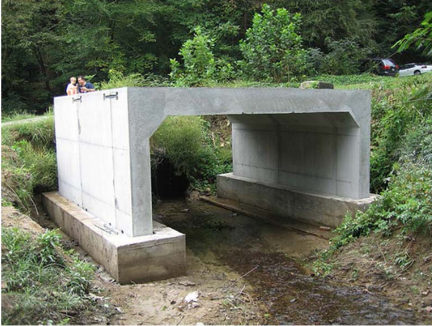
Example of Three-Sided Box Culvert (size and dimensions not to project specifications)
