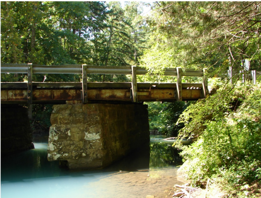
Existing Bridge with Stone Masonry Piers
